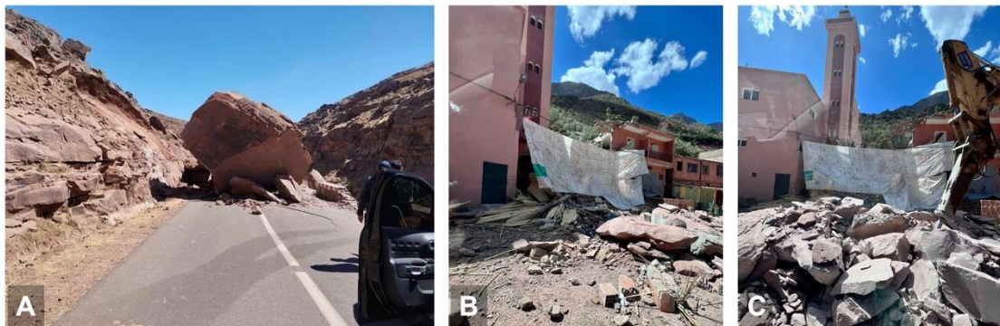
Fig. 6. Impacts of the 8 September Earthquake in the High Atlas Mountains. A) Boulders blocking a road (probably near Okimden about 40 km S of Marrakech, 11 September 2023). Source: Maroc Defender (@Empirechrifien1). https://twitter.com/Empirechrifien1/status/1700845696864117238 . B and C) Landslide deposit (aggregation of rock blocks) that destroyed buildings, photographed along the canyon from Ourika to Siti Fadma (11 September 2023).
