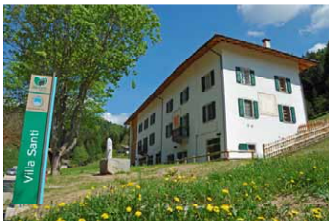
Fig. 2 – Villa Santi, Park house restored following principle of energy conservation.
