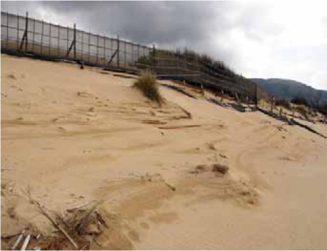
Fig. 5 – Windbreaks in the Buggerru dune, building to prevent sand dune drift onto near road.
