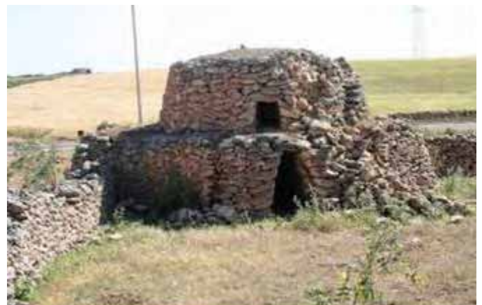
Fig. 6 - Tazotas, dry construction characteristic of Doukkala
