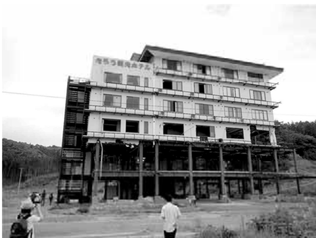
Fig. 5 - Taro Kanoko Hotel, which escaped tsunami of 11 March 2011 in Miyako city, Iwate Prefecture. Tsunami reached up to the third floor of this hotel and washed away all houses around it. It stands within the area protected by a 10m high embankment. Photo taken in August 2012.
