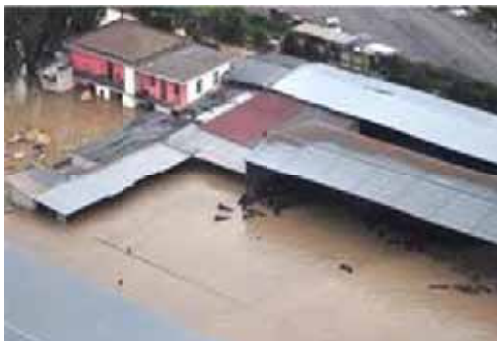
Fig. 2 – Flooding of River Sele:buffalo farm.
