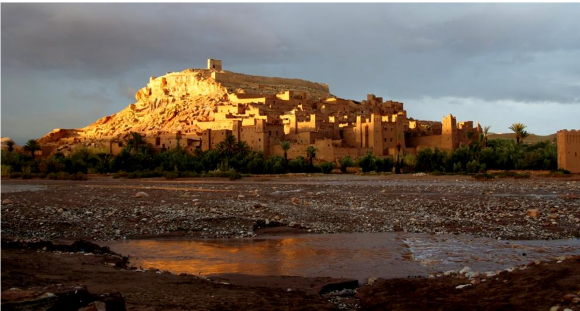
Fig. 3. Ait Ben Haddou Kasbah, an example of a traditional architecture of a pre-Saharan habitat.
