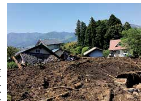
Landslide caused by earthquakes at Minami-Aso village
